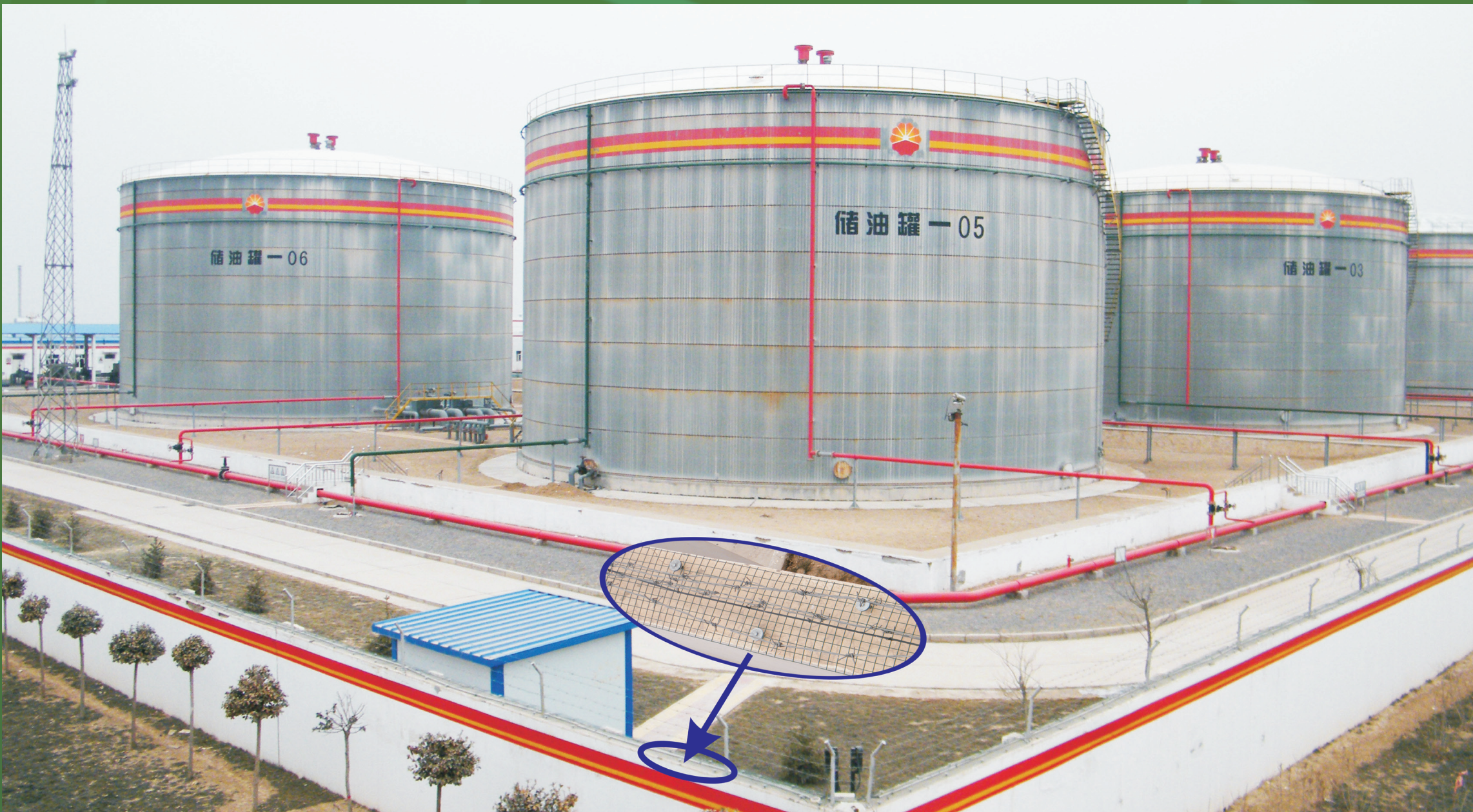
Perimeter security and oil pipeline protection application
