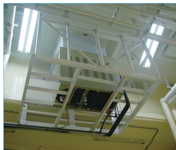
示範裝置：夜間電蓄冷微膠囊相變材料蓄能裝置 Prototype: MPCM slurry storage of night time electric cooling
